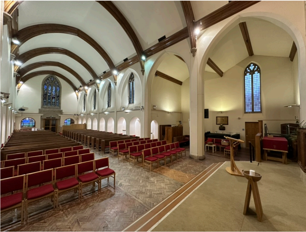
Photo 9 – The Nave & North Transept viewed from the East Chancel
