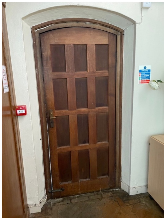
Photo 7 – The door in the East wall of the South Transept
