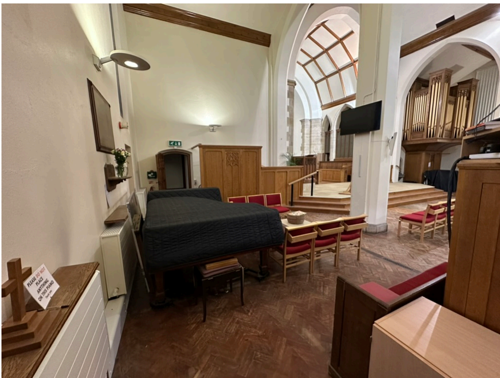
Photo 14 – North Transept viewed from its South-West corner
