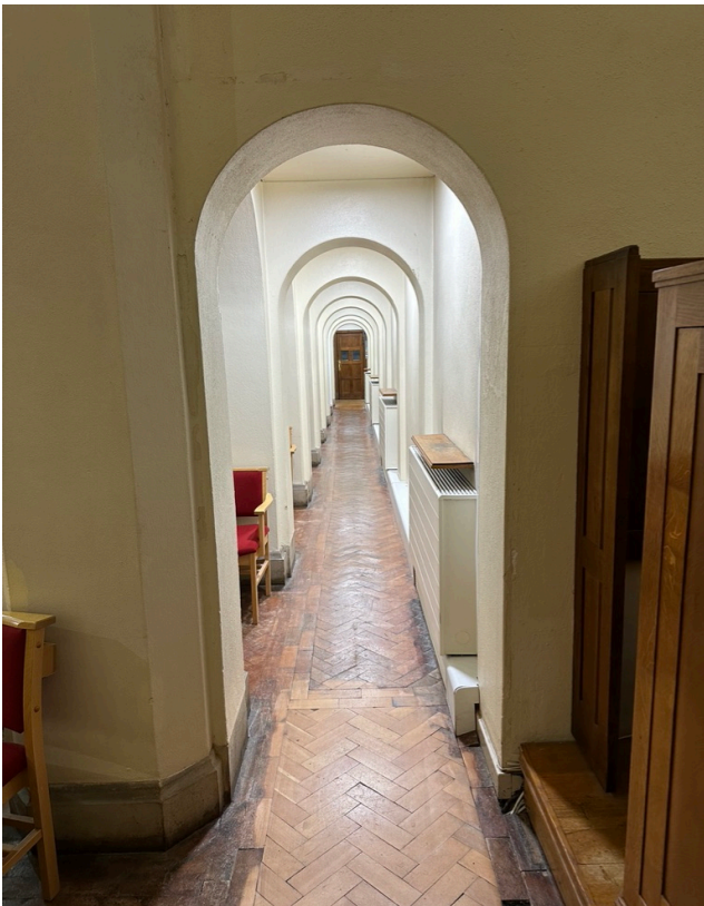
Photo 18 – North Colonnade viewed from the East end
